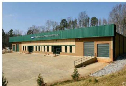
Our Distribution Center
